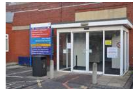
24 Vickers Courtyard Access to Vickers Corridor and wards
