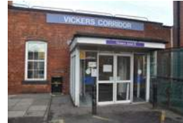
20 Access to Vickers Corridor and wards
